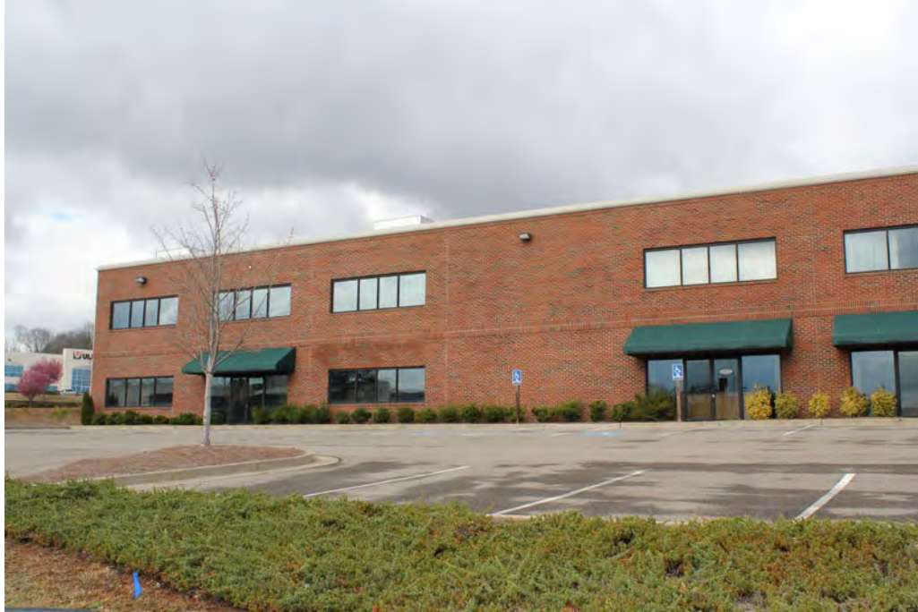
Picture 48—Blighted/Vacant Industrial Property
