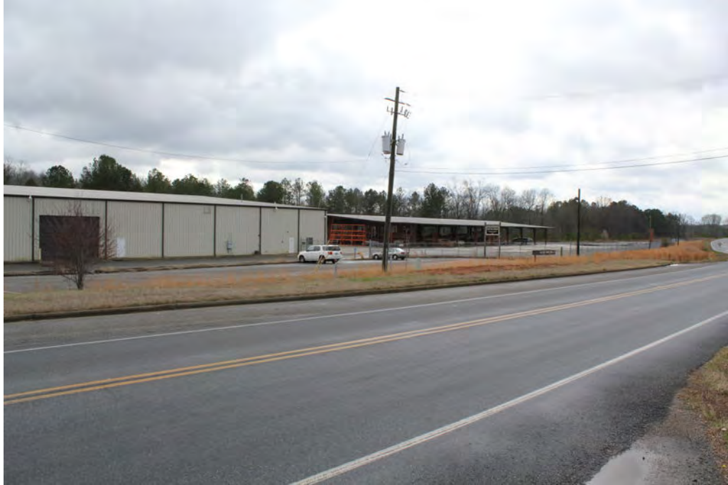
Picture 14—Blighted/Vacant Industrial Property
