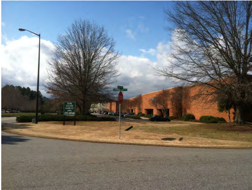
Picture 39—Blighted/Vacant Industrial Property
