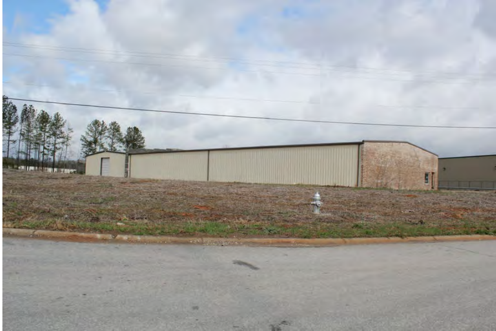
Picture 11—Blighted/Vacant Industrial Property
