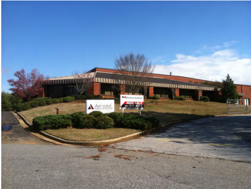
Picture 41—Blighted/Vacant Industrial Property
