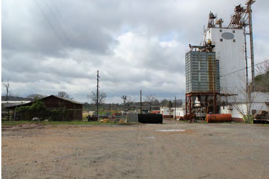
Picture 4—Blighted/Vacant Industrial Property
