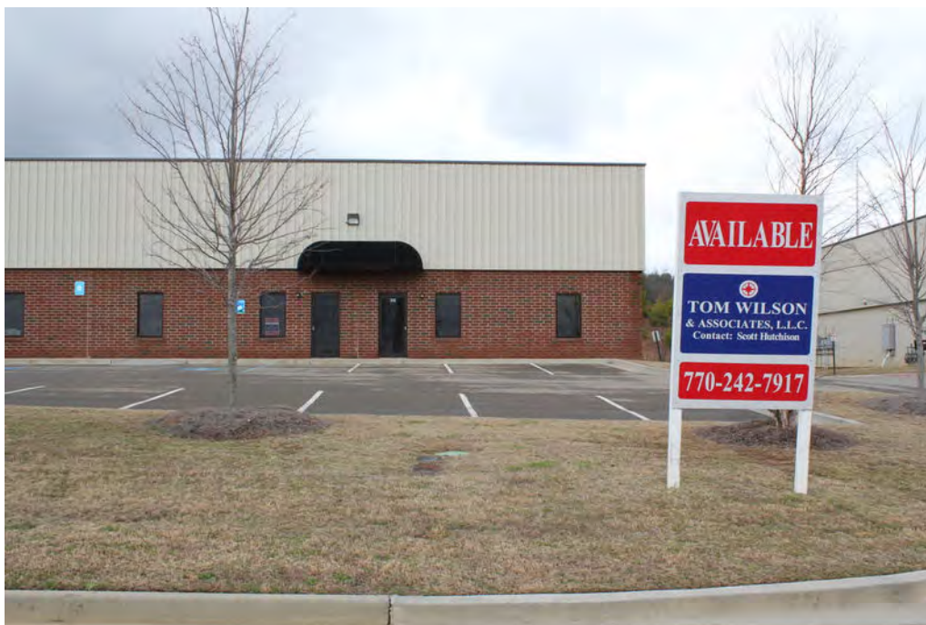
Picture 46—Blighted/Vacant Industrial Property
