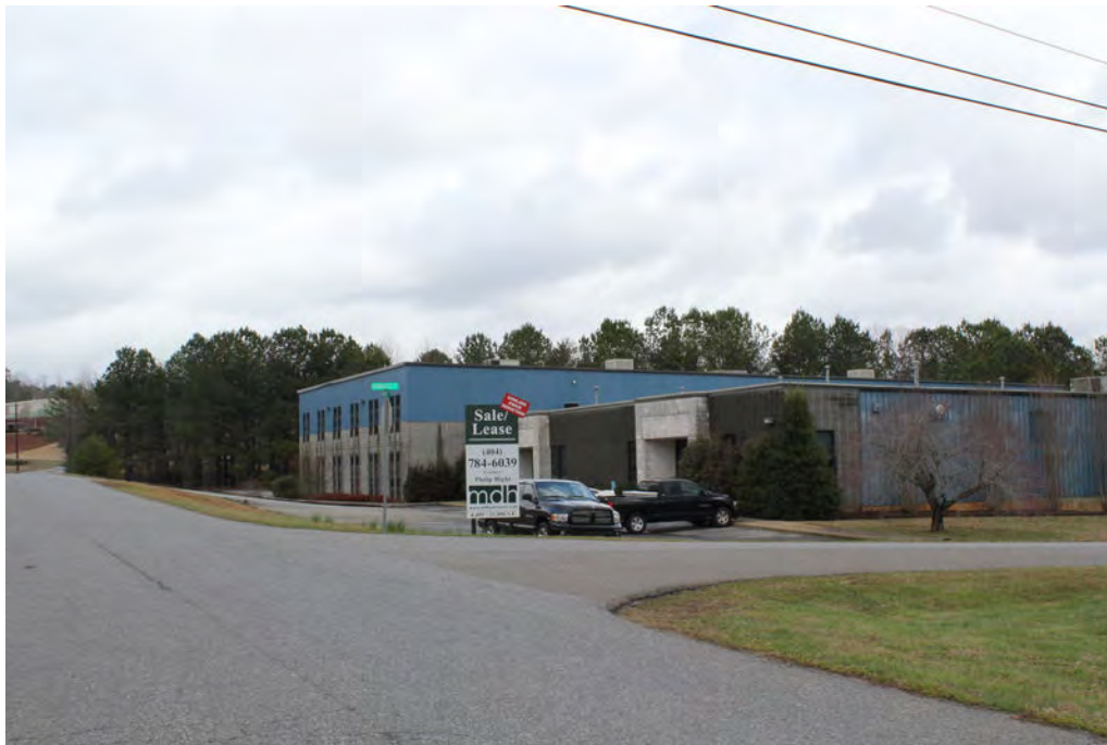
Picture 44—Blighted/Vacant Industrial Property
