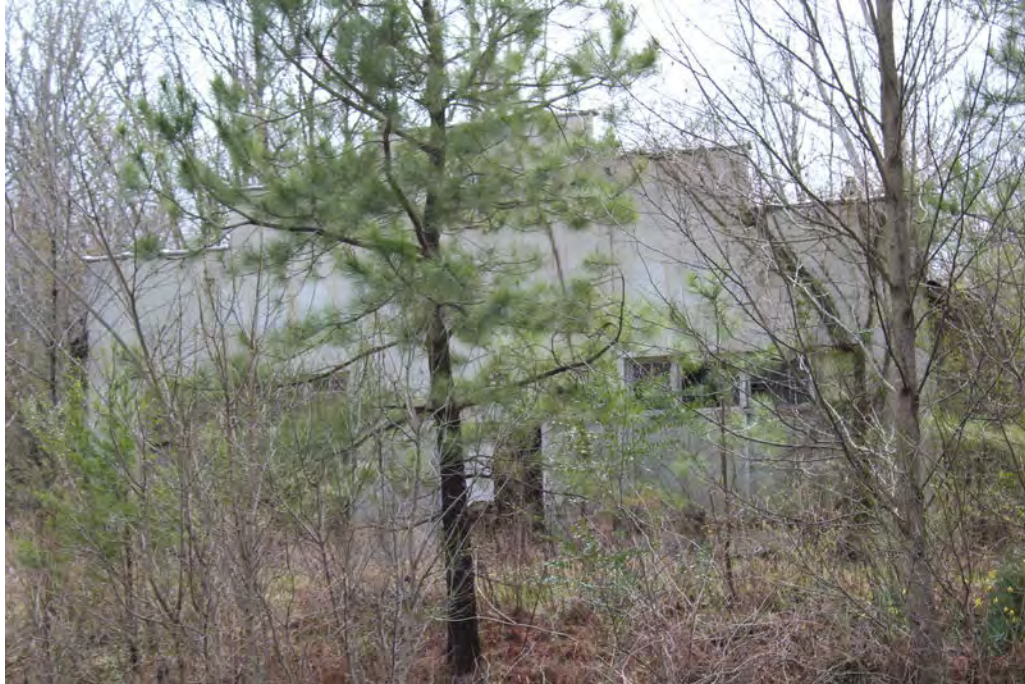
Picture 8—Blighted/Vacant Industrial Property
