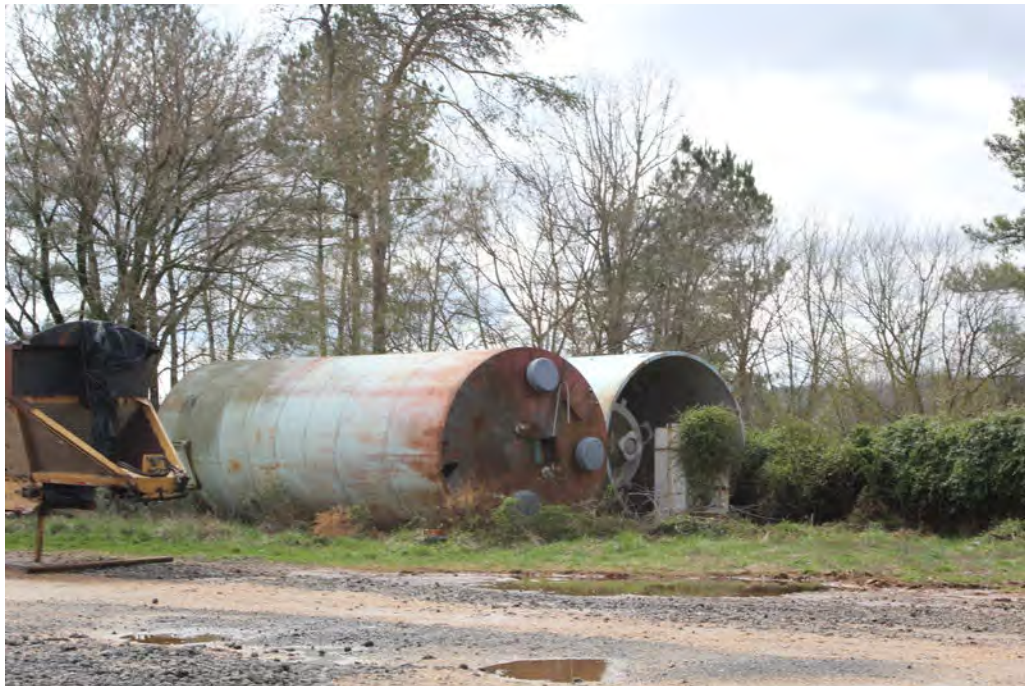
Picture 7—Blighted/Vacant Industrial Property
