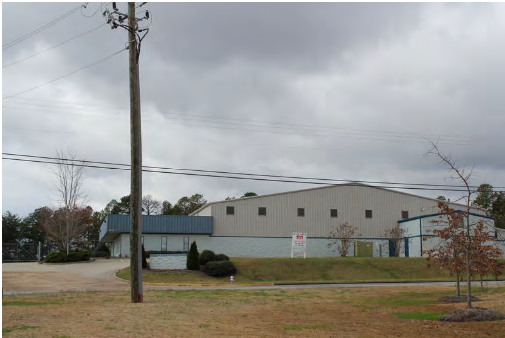
Picture 43—Blighted/Vacant Industrial Property
