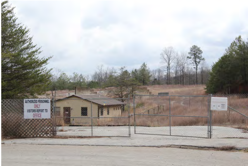
Picture 10—Blighted/Vacant Industrial Property
