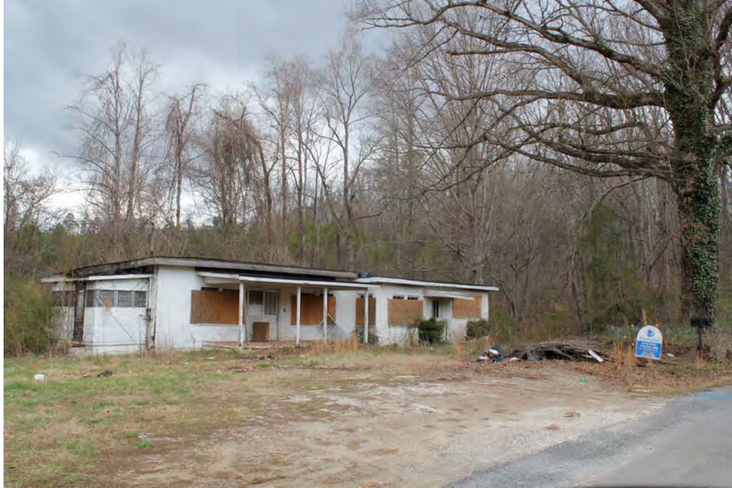
Picture 28—Blighted/Vacant Residential Property
