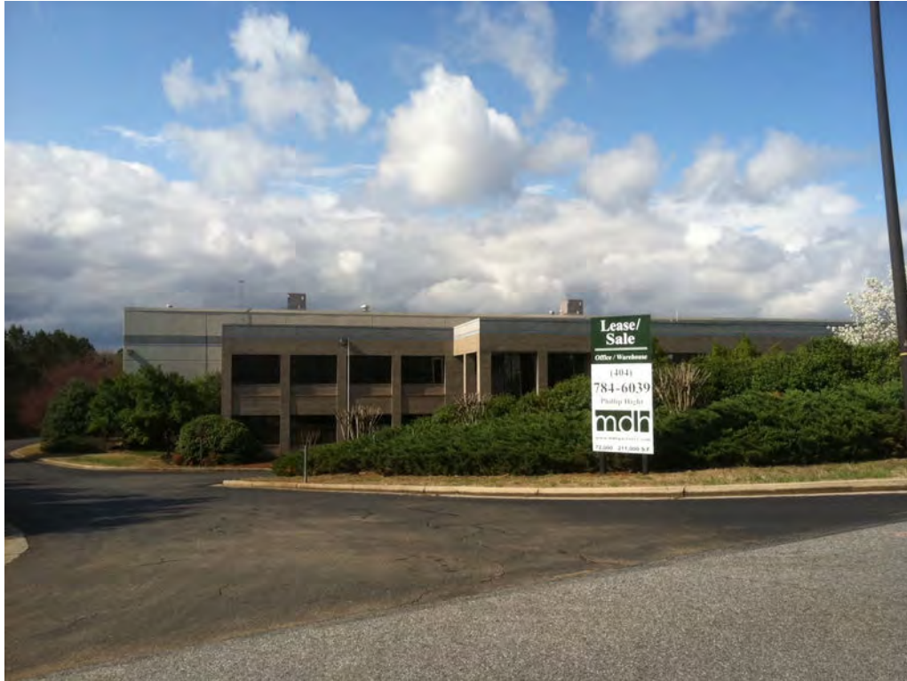
Picture 40—Blighted/Vacant Industrial Property
